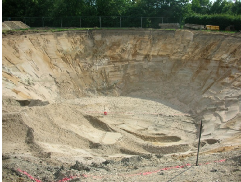
FIGURE 1.28 – Excavation du PTES de Eggenstein-Leopoldshafen[40].
